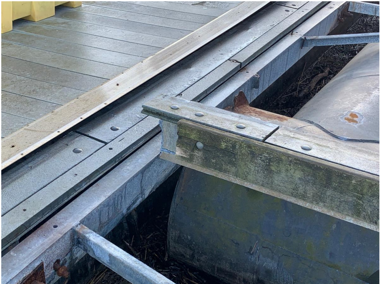
Broken side section on walkway pontoon
