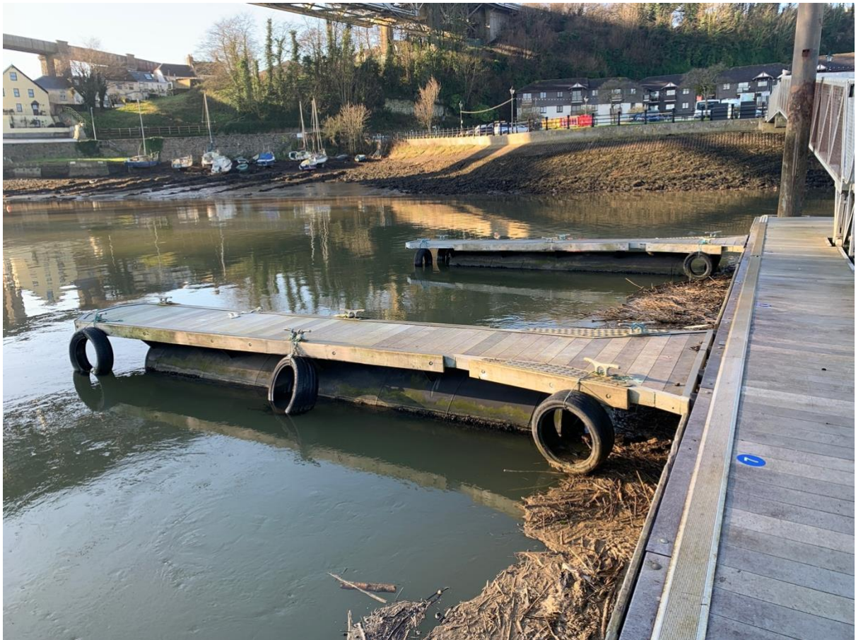
Finger pontoon links look unaffected but should be checked
