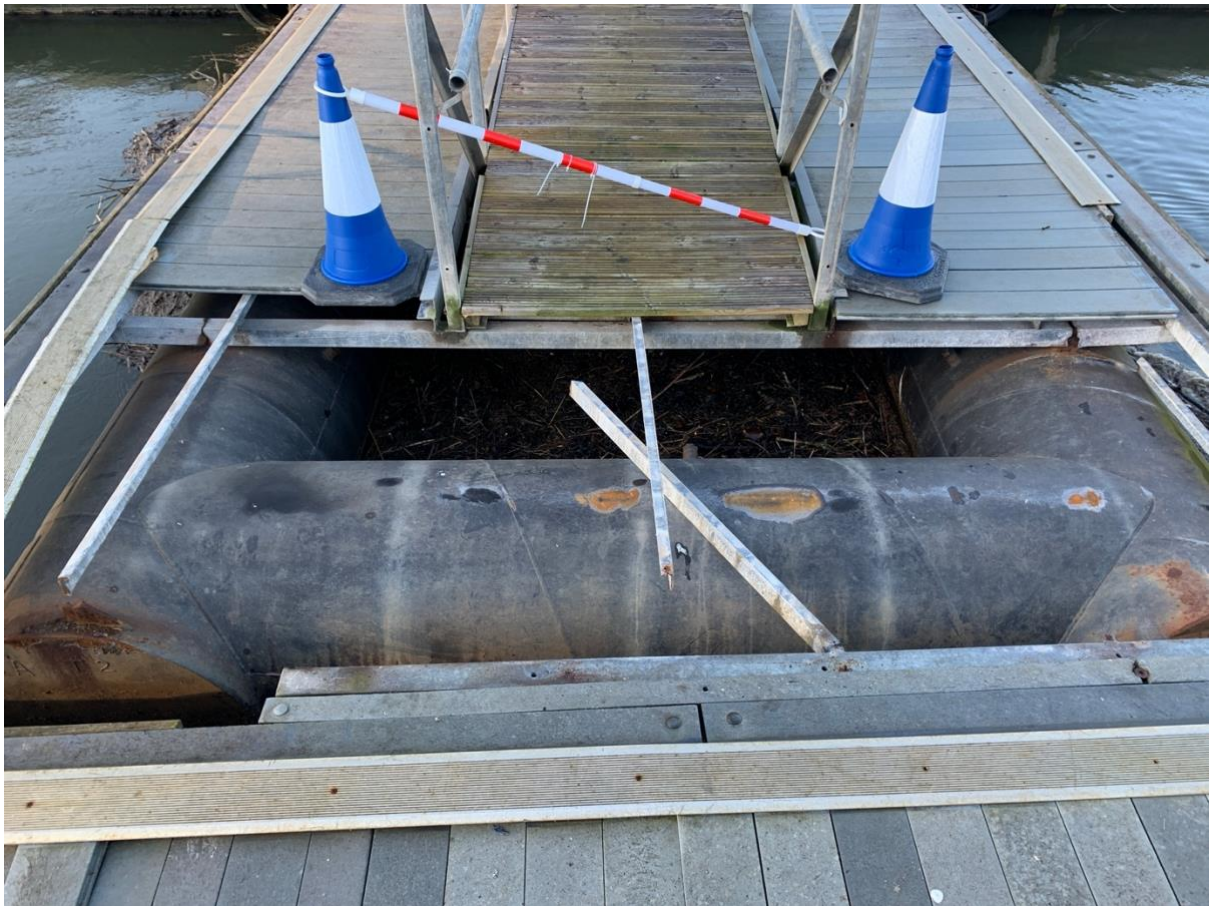
Damage at end of walkway pontoon
