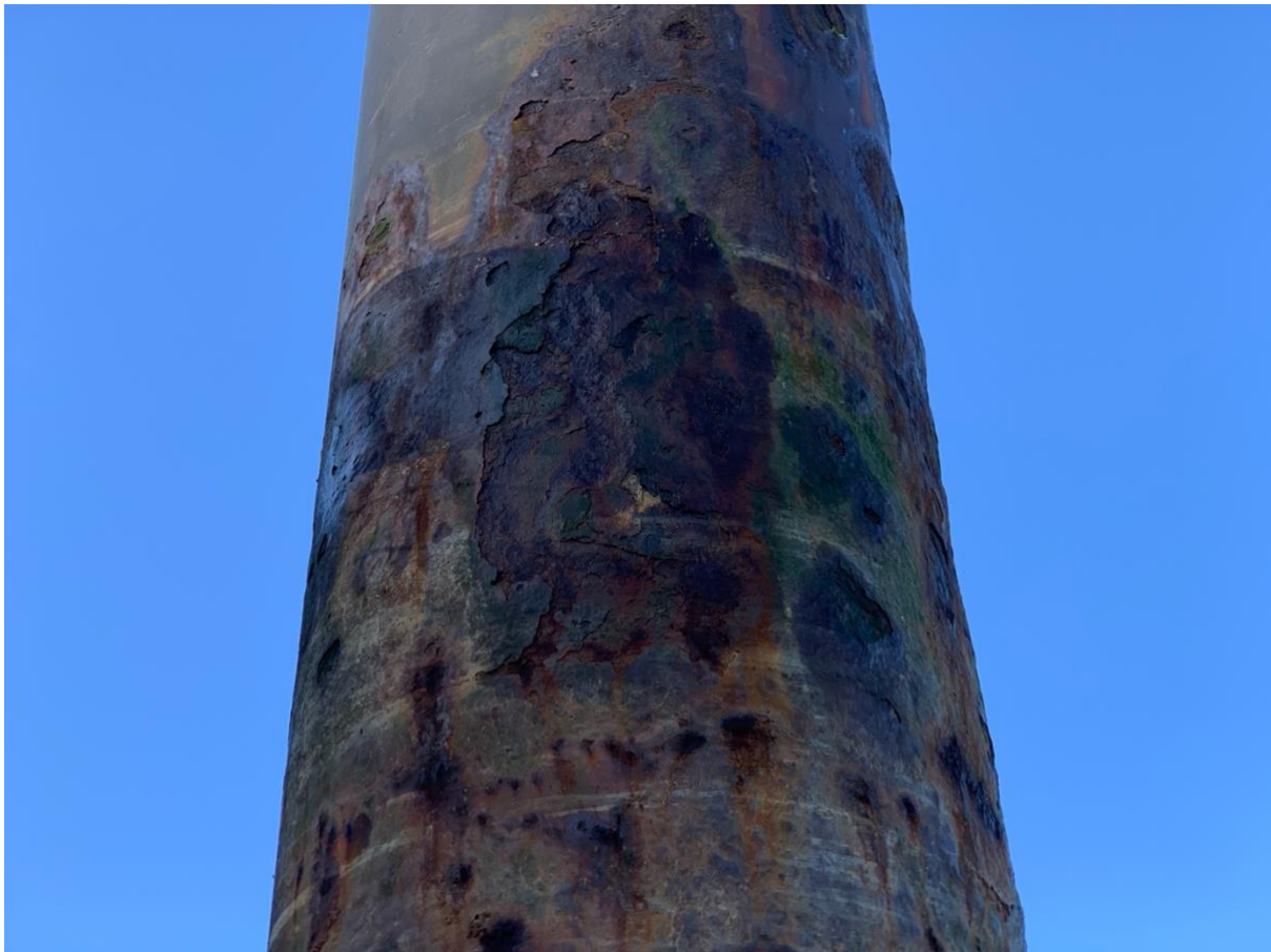
Pile corrosion
