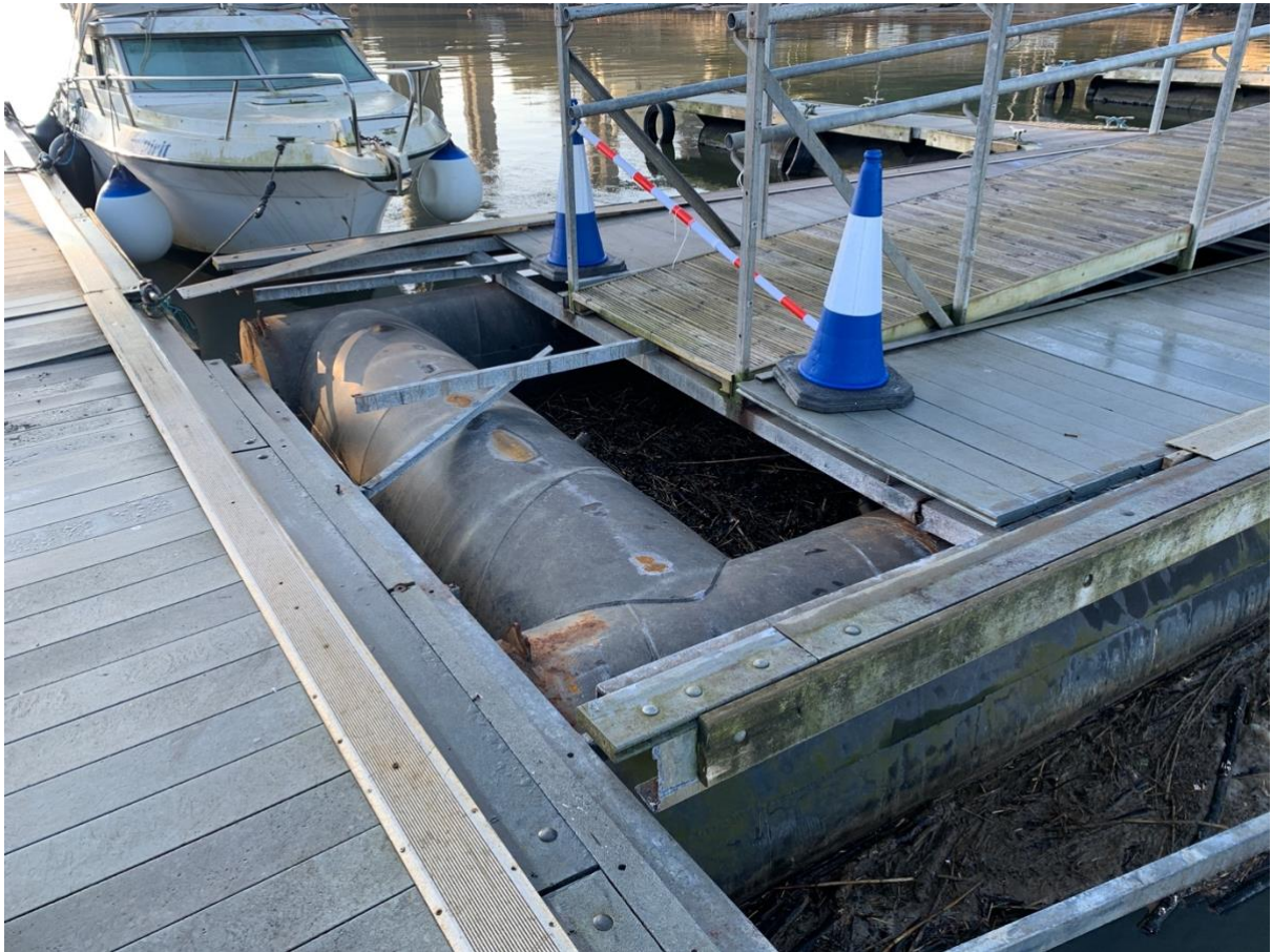
Damage at end of walkway pontoon
