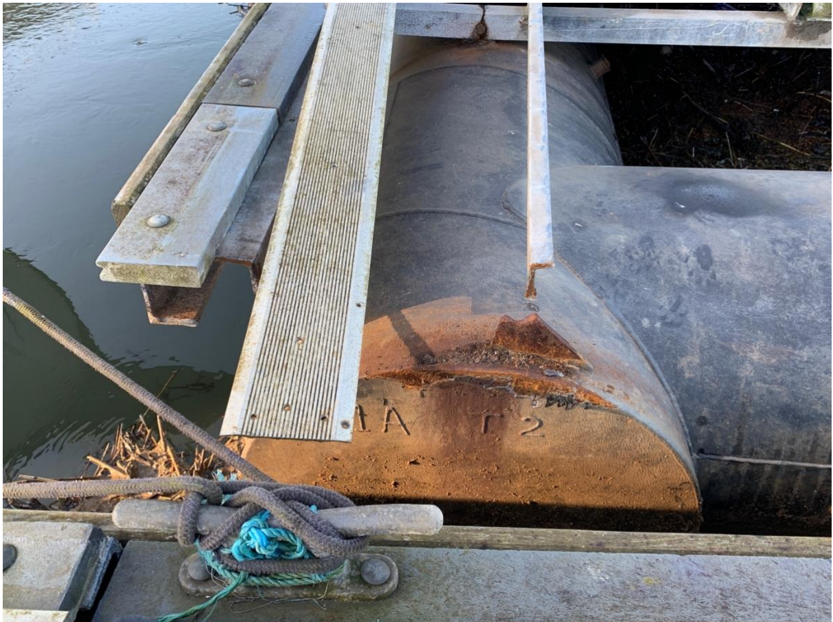
Broken side section on the other side of the pontoon.
